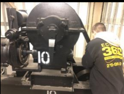
Vertical Transportation Pulley Maintenance
